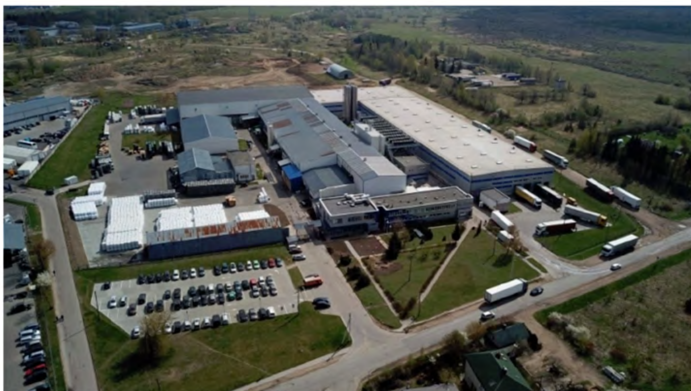
RETAL plant in Lentvaris, until February a 1,4 MW rooftop plant will be installed.
