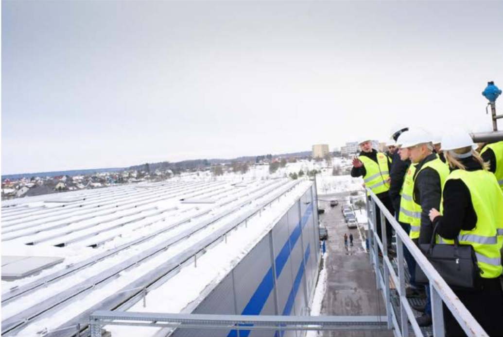
(Photo: The largest photovoltaic installation in the Baltics on top of the RETAL factory in Lentvaris, Lithuania. Credit: Tomas Lukšys)
