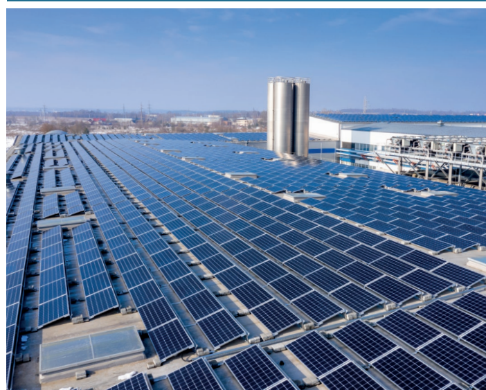
RETAL Lithuania photo-voltaic installation
